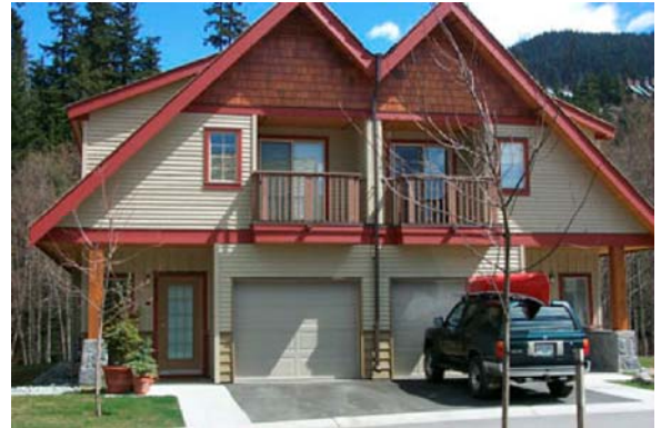
These three-bedroom duplex units, near Whistler's commercial area, are examples of housing that is restricted in resale price and occupancy.
